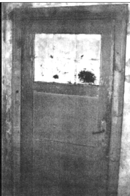
Illustration 2: One of the three doors of an alleged NS gas chamber for the execution of hundreds of persons at once with Zyklon B (hydrogen cyanide) (Krematorium I, Auschwitz, Poland, beginning of the 40's). This door is neither sturdily constructed, nor air-tight (e.g., the keyhole). It is partly glazed and opens inwards, i.e., into the room, where allegedly corpses were piling up.
