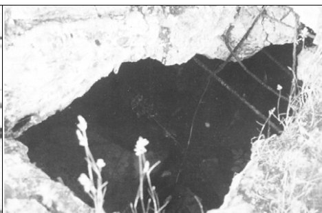
Illustration 6: Alleged Zyklon B input hatch in the roof of mortuary 1 (‘gas chamber’) of crematorium II; entrance to part of the cellar still accessible today.
